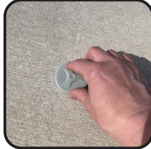
STEP 2 Twist in CAP-IT finger-tight only (Clockwise direction)
