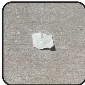
STEP 1 Cover CAP-IT with piece of masking tape
