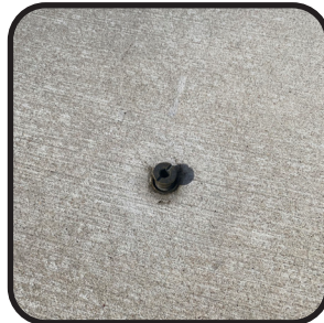
STEP 2 Install Anchor Stud to accept winter cover
